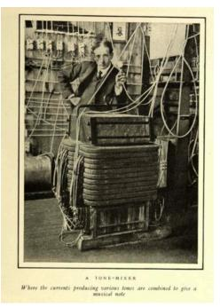
The article was written in 1906 and highlights the unique and extraordinary aspects of the Dynamophone (also called the Telharmonium) from the authors perspective. Numerous photos are included, from what the inside of a Dynamophone looks like, including samples of inductors and the wires, to images of Dr. Cahill himself.
