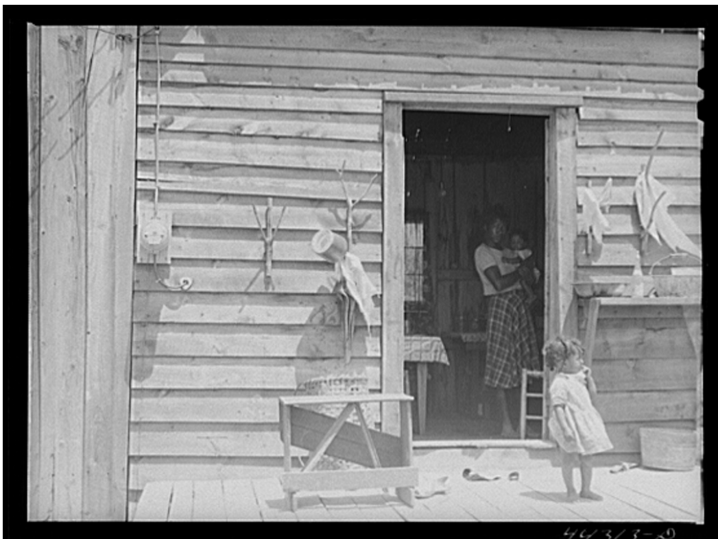
Delano, Jack, photographer. Negro tenant farmer's house showing REA Rural Electrification Administration electric meter on wall. Greene County, Georgia, United States, May 1941. Photograph. https://www.loc.gov/item/2017794691/ . Accessed 4 June 2018.
