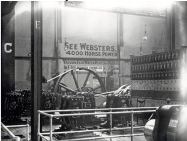
Arc System Generator
