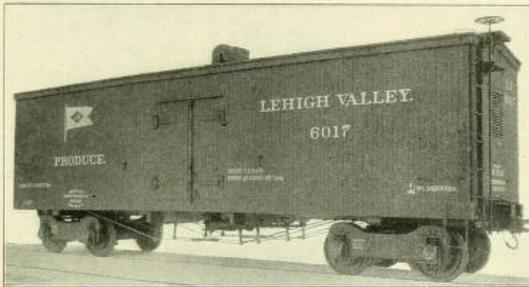
Fig. 9. Produce Car. Capacity, 60,000 lbs. Weight, 38,500 lbs. Length, 34 ft.
