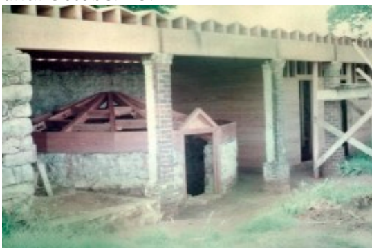
The ice house roof under reconstruction in the 1950s.
